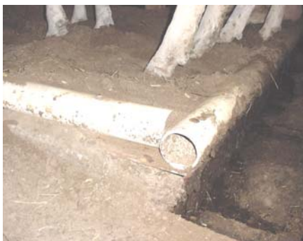
Photo 2: John Nortz design: a steel plate carrying the PVC pipe hangs over the gutter to maintain the bed length.
