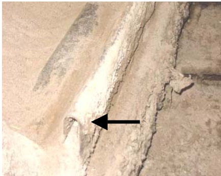
Photo 1: Ernie Beyer purchased this retainer – 3 in. high and 1.25 in. wide at the top. The base is lagged to the concrete stall base.
